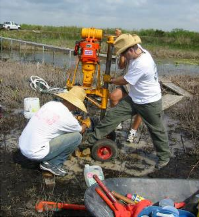
Installed groundwater monitoring wells at an average depth of 1.34 m on the islands and ridge and slough
